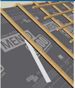
Remove the backing strip from the TESCON NAIDECK tape as vertical battens are installed over top of joists. Add cross battens for metal or tile roofs.
