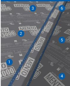
Overlap additional sheets of MENTO, working up one side of the valley to the roof ridge, extending each membrane approximately halfway into the field and sealing with TESCON VANA tape. Then on the opposite side, repeat from bottom to top.
