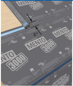
Unroll the next row of membrane and align by using the printed guides - overlap the bottom sheet a minimum of 6". Use the printed markings as a guide. Activate the integrated adhesive strips by removing the release papers and pressing down on the connection with a PRESSFIX, roller, or your hand.
