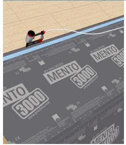
Only secure the membrane in areas that will be below an overlap, below battens and TESCON NAIDECK, or taped with TESCON VANA.
