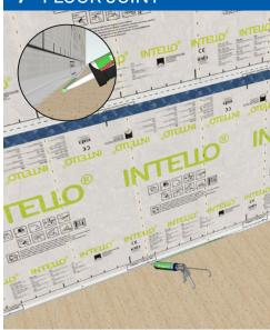
Apply CONTEGA HF adhesive on the floor board, forming a continuous bead approximately 1/4" thick. Lay the membrane in the adhesive bed, leaving an expansion joint. Do not press the adhesive completely flat.
