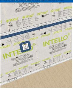
Use INSTAABOX to create an airtight cavity for light switches and electrical outlets when there is no service cavity. Tape INSTAABOX to the membrane with TESCON VANA.
