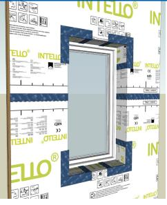
Use rectangles of INTELLO to cover exposed rough opening sheathing and staple into place. Airseal these patches with TESCON VANA tape to the surrounding membrane. Press tape firmly with a PRESSFIX.
