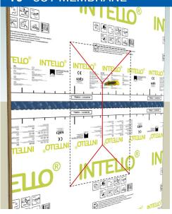
Cut the membrane from each of the corners of the rough opening towards the center at 45° angles. Then cut vertically down the center.
