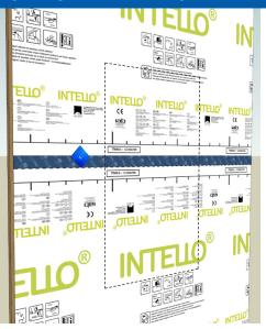
Install INTELLO on the interior of the wall per INTELLO installation instructions. Use TESCON VANA tape to airseal membrane overlaps. Use the dotted lines on ProClima membranes to align overlaps properly and as a guide to center the tape over the joint. Press tape firmly with a PRESSFIX.
