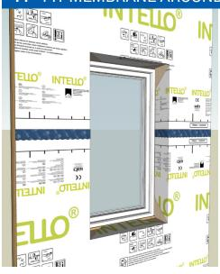
Fold back the edges of the membrane into the rough opening and secure by stapling.
