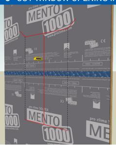
Cut along the top of the rough opening. Cut from the top corners of the RO at 45° angles up and away from the center. Cut down the center to the bottom of the RO, and then cut along the bottom edge of the RO.
