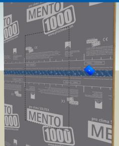
Install the WRB over sheathing per SOLITEX MENTO wall application instructions. Use **TESCON VANA tape** to airseal membrane overlaps. Use the dotted lines on ProClima membranes to align overlaps properly and as a guide to center the tape over the joint. Press tape firmly with a PRESSFIX tool.
