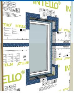
After installation of the L-shape pre-made corners, seal the window frame to the INTELLO. Apply narrow sections of TESCON/ CONTEGA tape to the frame - make sure to work bit by bit - so tape will not be applied to parts of the frame that won't be covered by trim/ drywall. Remove wide release strips from the tape and apply firmly to INTELLO. Ensure there is at least a 1" overlap of tape connections.
