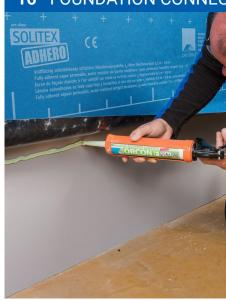
When sealing to rough substrates such as concrete components, apply a line of the CONTEGA HF adhesive with a thickness of at least d = 3/16" (5 mm).
