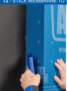
Once ADHERO has been cut out, fold it onto the soffit and adhere it in place.
