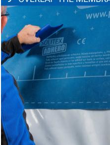
Apply all the remaining membranes - one by one - horizontally in an overlapping, waterproof manner.
