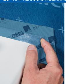
Seal angular penetrations using TESCON PROFECT tape.
