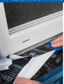
Apply window sealing tapes (e.g. CONTEGA SOLIDO SL on the inside and CONTEGA SOLIDO EXO on the outside) to the blind frame all around the window.
