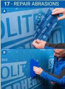
A. Adhere TESCON VANA tape in widths of 6" or 8" (150 or 200 mm) over any defects in ADHERO.
