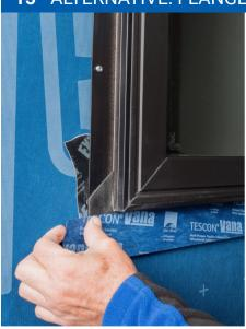
Insert the window, fasten it and the seal with TESCON VANA on ADHERO all around the window in a waterproof manner.
