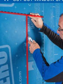
The membrane is first adhered over any window openings.
