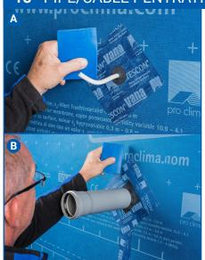
A. Seal pipe feedthroughs with a suitable ROFLEX gasket. Adhere the gasket to the subsurface using TESCON VANA tape. Smooth adhesive joints firmly with a PRESSFIX.
