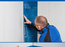
For interior corners and, if necessary for exterior corners too, cut a strip of ADHERO that is at least 16" (400 mm) in width and adhere it in place with equal parts on each of the walls.
