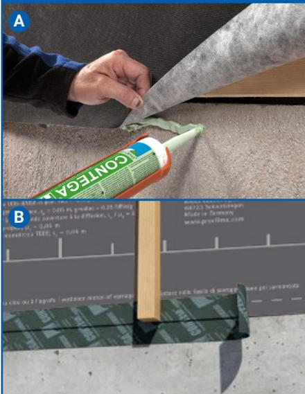
A. Use CONTEGA HF to connect to concrete foundation, or other rough surfaces. Make sure substrate is stable or use TESCOIN PRIMER RP. Apply a 1/4" (6mm) wide bead (wider on rough surfaces). Press the membrane into bead, with room for expansion/contraction of structure. Do not press adhesive completely flat. Let cure for 48 hrs.
