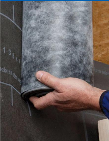
After the first layer is applied begin the second row. Use the printed markings as a guide and shiplap the WRB by 6" (150 mm).
