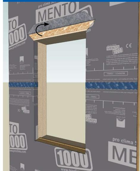
Fold up upper part of membrane and temporarily hold in place with masking tape. This is so it can be installed over the header flange of the window later.
